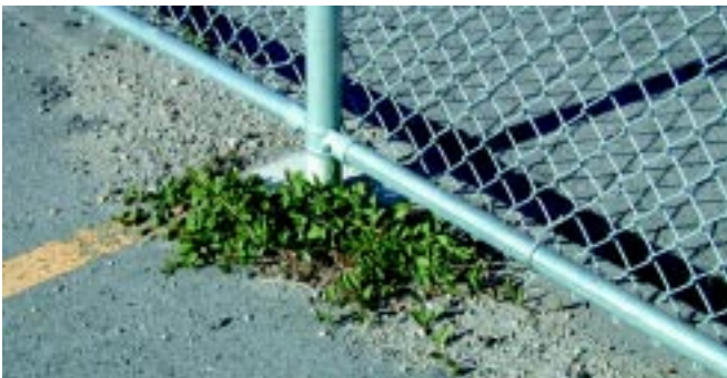
Weeds quickly invade openings in paved surfaces and can speed degradation of these surfaces.
